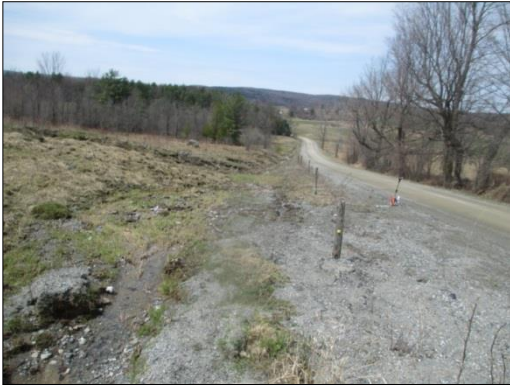
BEFORE – Unstable road and ditch. Photo credit: MRBA
