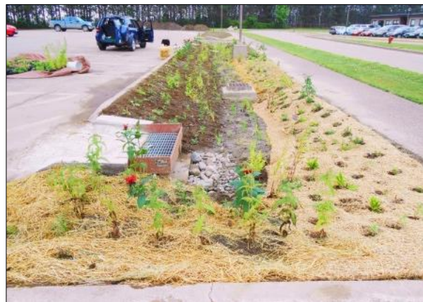
AFTER – School parking area after installation of bioretention system. Photo credit: Lamoille County Conservation District
