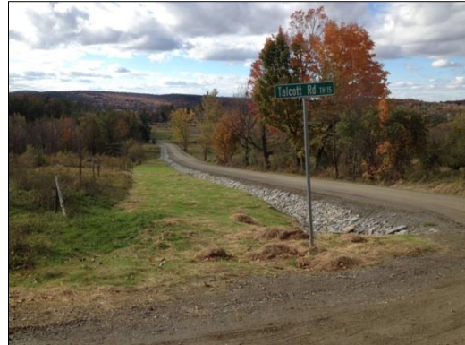
AFTER – Stabilization of eroding road and ditch and livestock exclusion with fencing. Photo credit: MRBA
